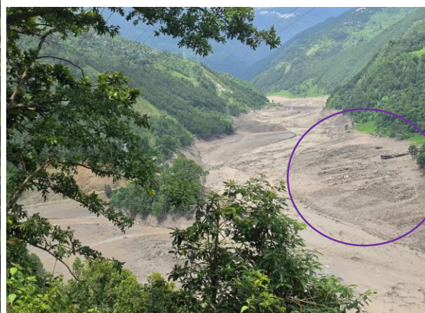
Everything swept away after the flood
