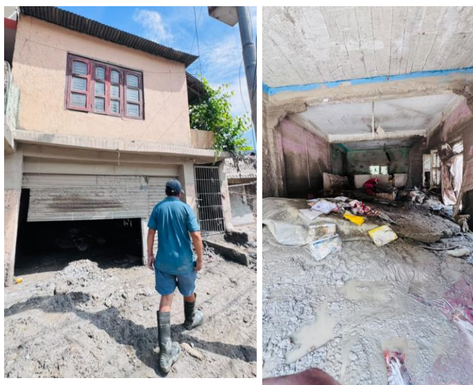
Bipin Malla's residence filled with flood debris.
