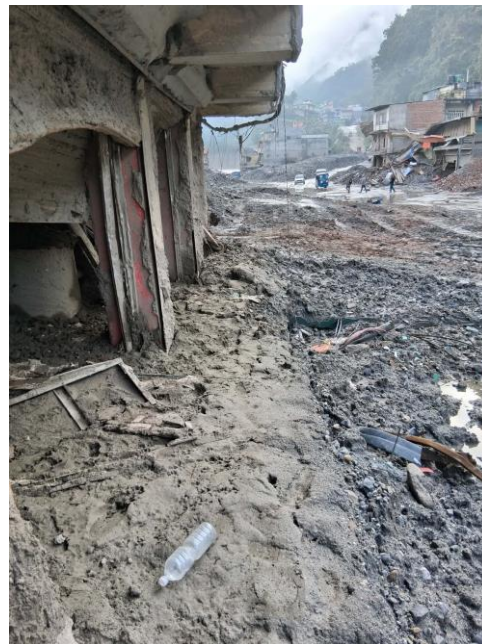
Residence and media archives covered with flood debris
