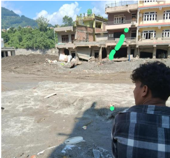
Kiran Adhikari's residence marked with green spots flooded
